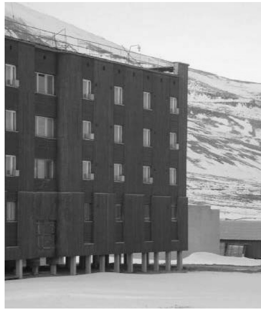
Fig. 10. Housing in Pyramiden. Foundation: reinforced concrete piles.
