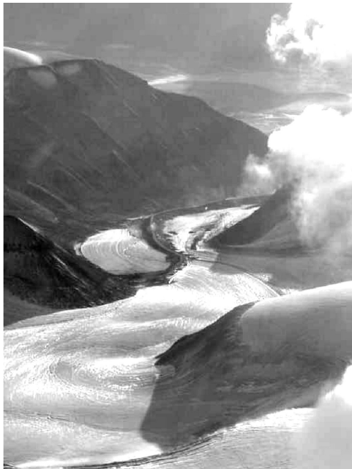
Fig. 14. Road on the Høganäs glacier from Sveagrava to the new mine, utilizing a mid-moraine as foundation for the road embankment.
