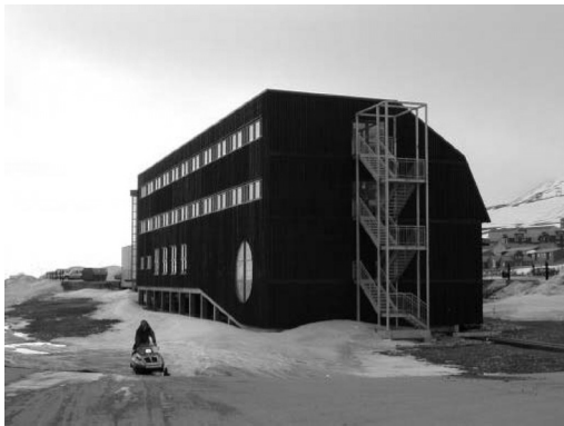
Fig. 9. University Centre in Svalbard, Longyearbyen. Foundation: excavation, replacement and concrete footings.
