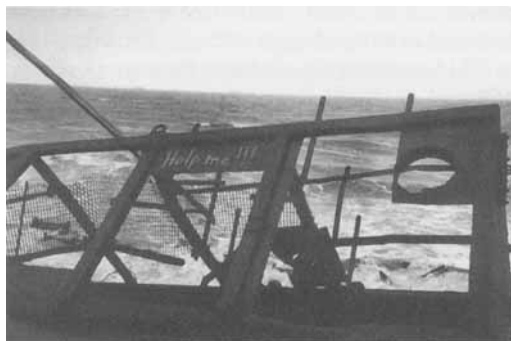
Fig. 3. Crumbling coast of New Varandei. Photo: A. Golovnev.
