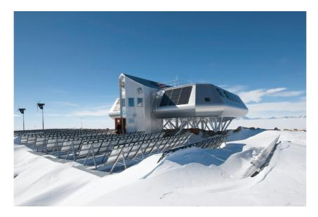
Fig. 1 Princess Elisabeth Antarctica, with some of the solar photovoltaic panels and wind turbines that power the station.
